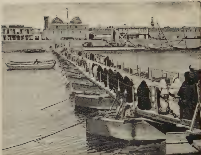
The new boat-bridge across the Tigris at Bagdad, from the east. Two pontoon bridges connect old Bagdad with the newer suburbs on the east bank.
